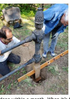
2. Many of the 20 foot square lots in the cemetery are outlined either with a concrete curbs or a metal fences. Both styles can fall into disrepair through weathering or damage. One such lot is in the southeast corner of the grounds. Several handsome cast iron posts support decorative iron pipes. Several years ago, one of the corner posts was damaged beyond repair. Through the generosity of Masonic Lodge #11, we have been given funds to create a new post.
