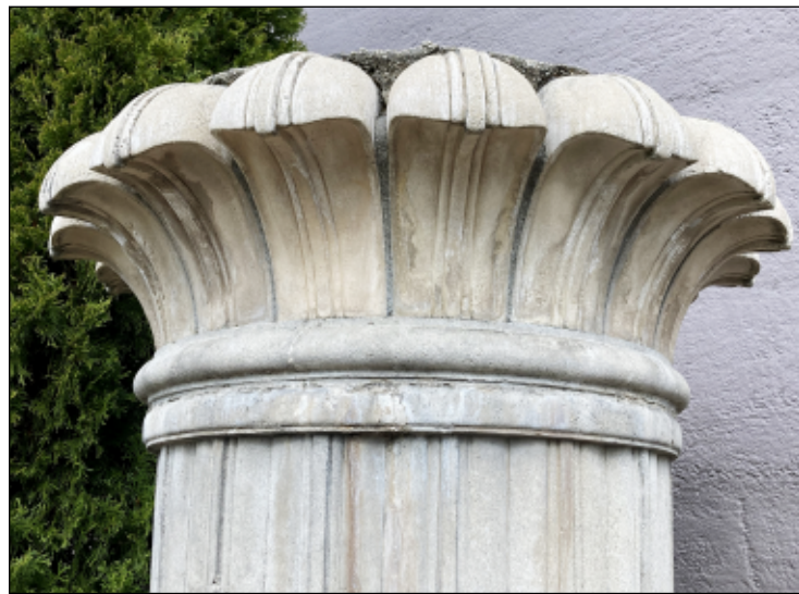
Entrance Vase after repair
