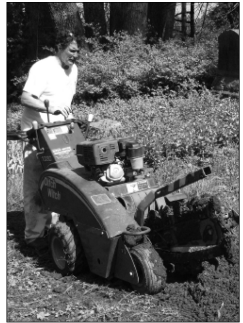
Trenching for water line installation
