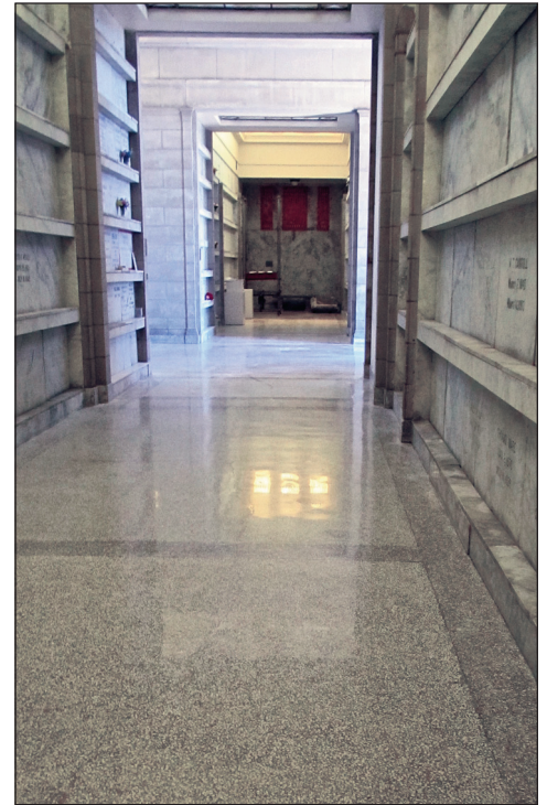
Terrazzo floor after
