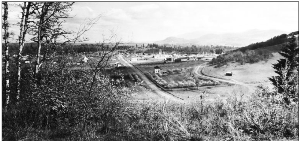
Early picture of Fairmount looking North
