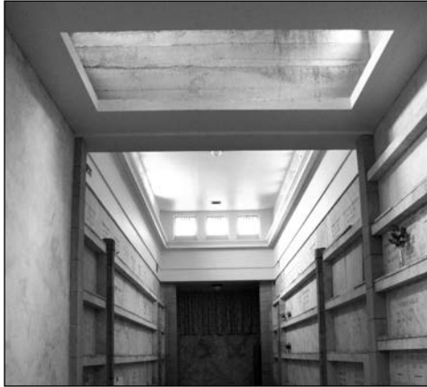
Hope Abbey ceiling before window installation
