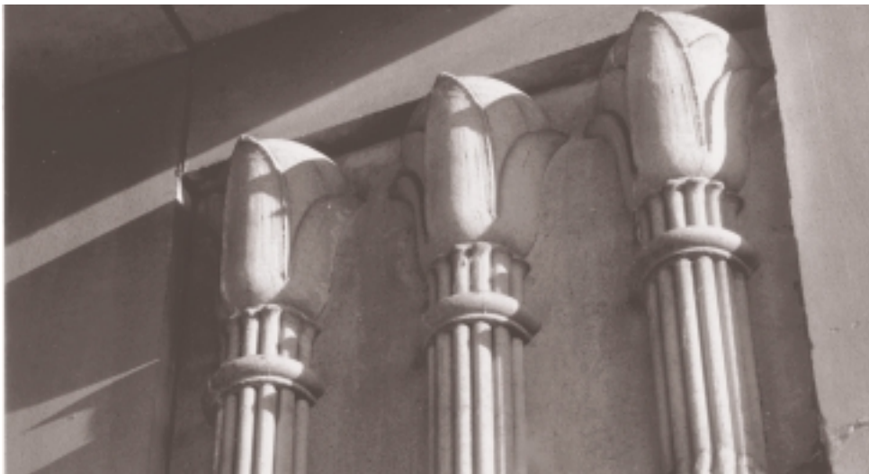
Above: Precast concrete detail from Hope Abbey Mausoleum, built 1913-14.
