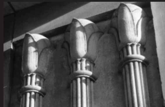
Precast concrete detail from Hope Abbey Mausoleum, built 1913-14.
